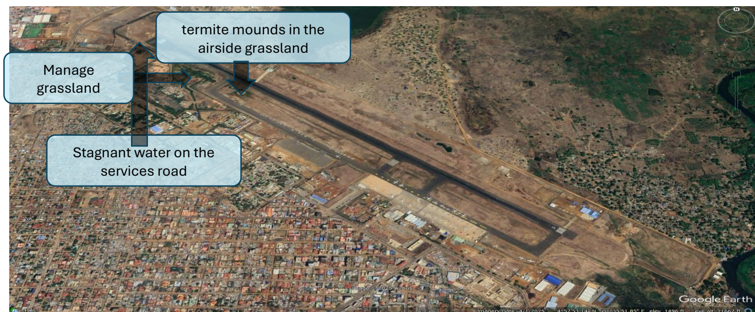
Figure 1: – On airport hazards
